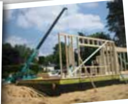
Timber Frame Work
